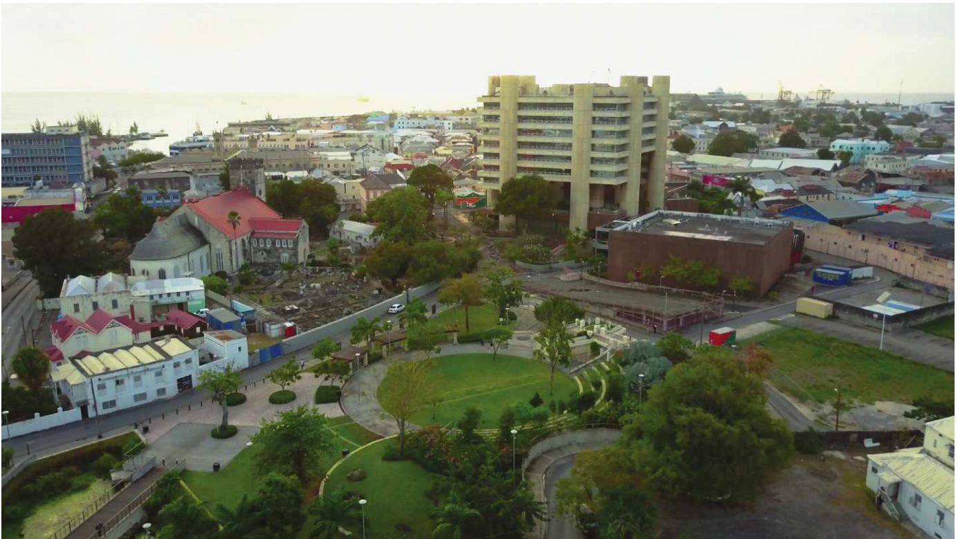
An aerial view of the Bank's headquarters and environs.
